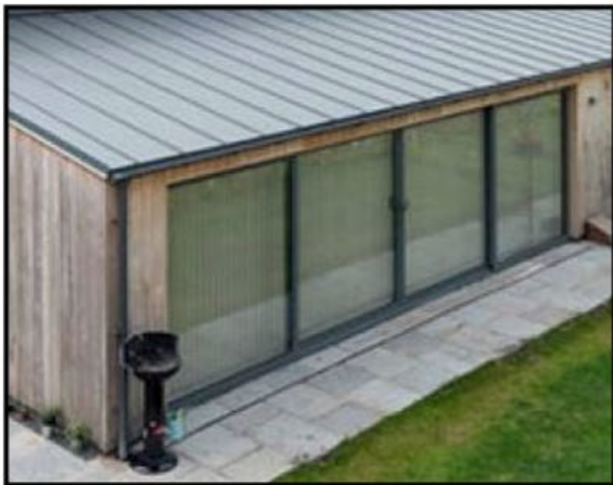
composite aluminium/timber windows ppc finish colour - anthracite
