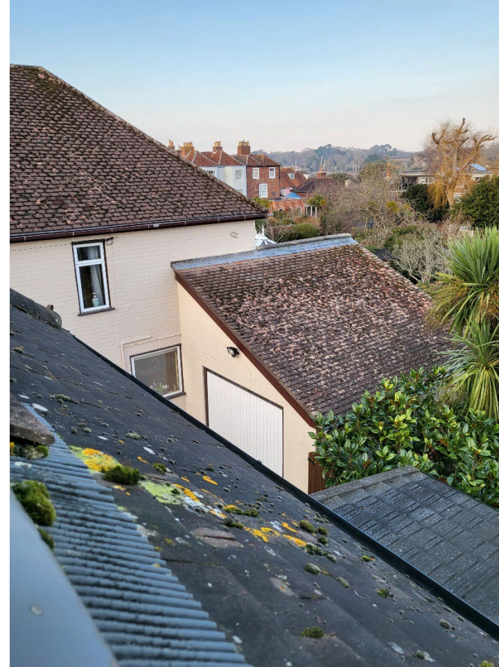
View from existing rooflight
