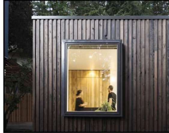
projecting bay window composite aluminium/timber windows
