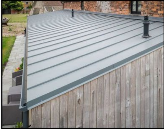
aluminium standing seam roof system ppc finish colour - anthracite
